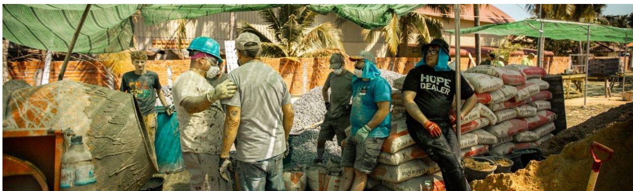
Laying block, welding roof steel, and working the mixing station under the shade cloth.
